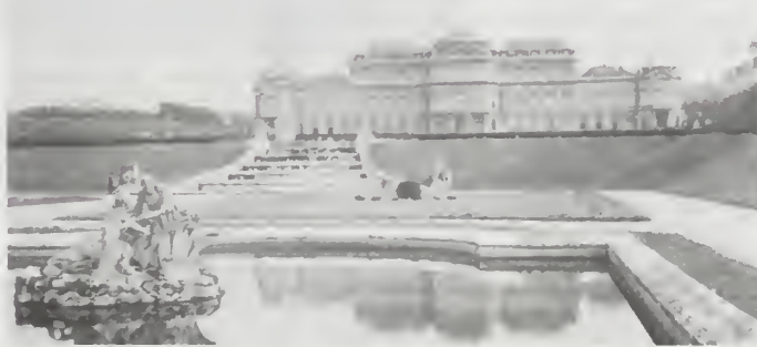
Garden facade of Belvedere Palace, Vienna, by Johann Lucas von Hildebrandt Foto Marburg—Art Resource/EB Inc
